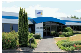
Standby Mercura in Blois u. Nantes, France
